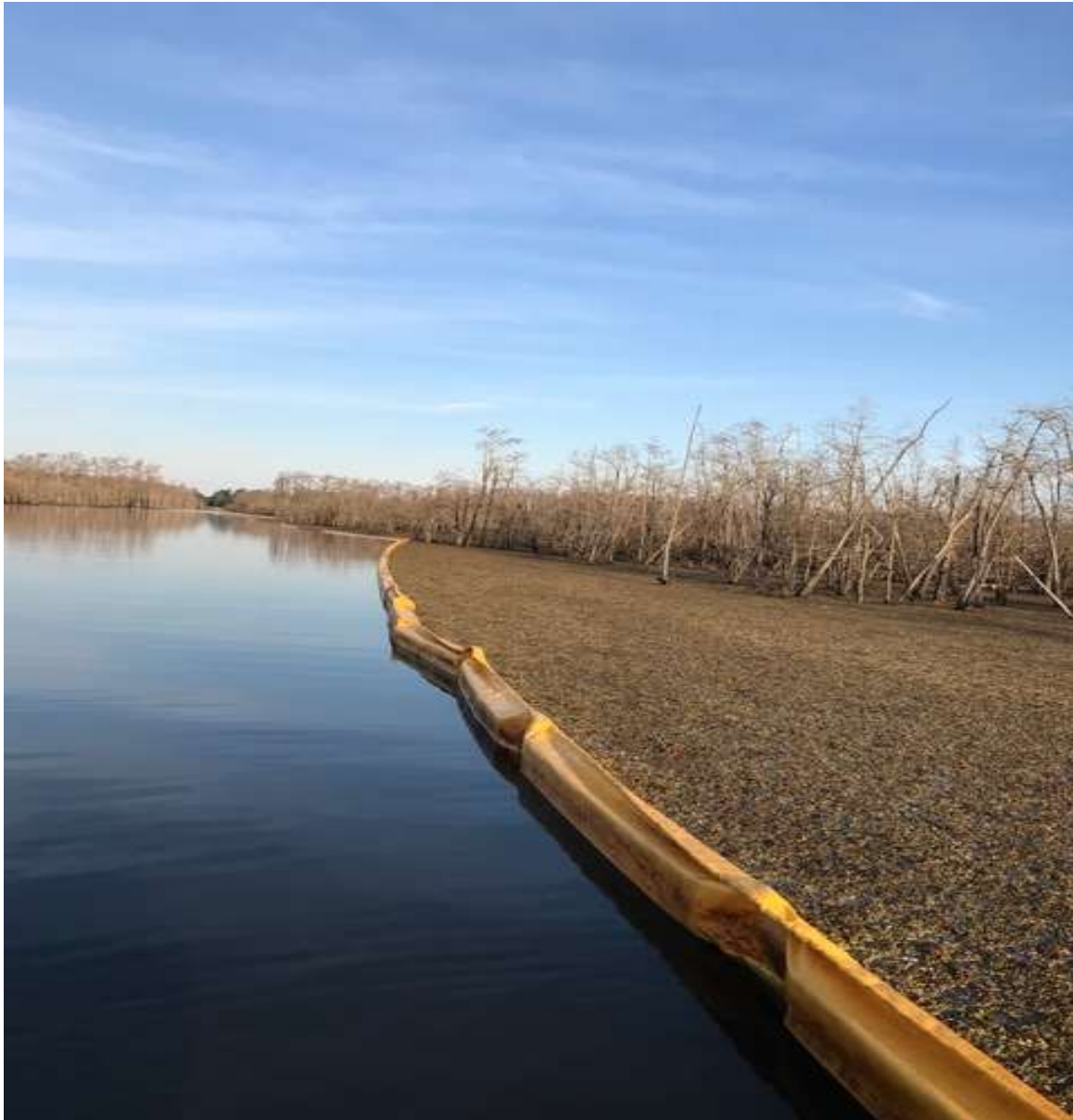
Figure 3. Four thousand-foot vegetation containment boom placed along North side of pipeline above Mulligan Inn Landing.
